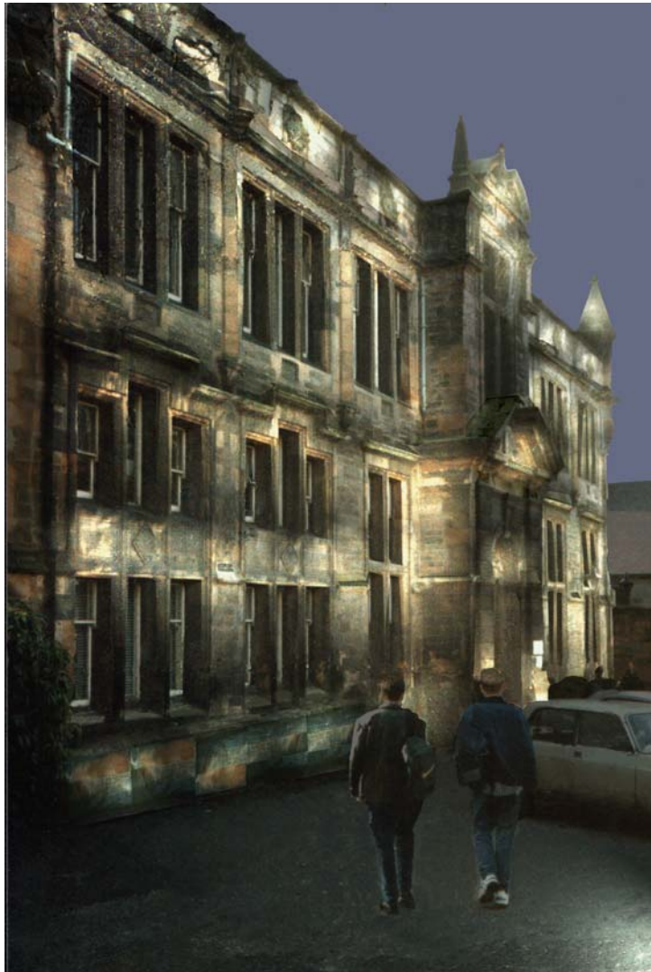
Floodlighting at the North Elevation.
